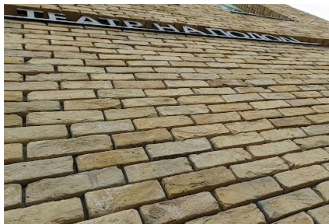
figure 6. Reused brick facade on the Theatre on Podil by Drozdov&Partners. Kyiv, Ukraine, Dec 2023
